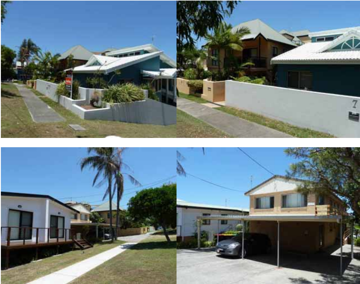
Properties at 7-13 Clarence Street, Yamba
