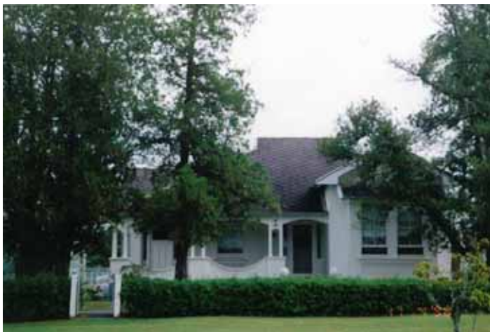
27 Orara Street Lot 1 DP 116480
